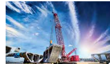
06 MANITOWOC CRAWLER CRANES
