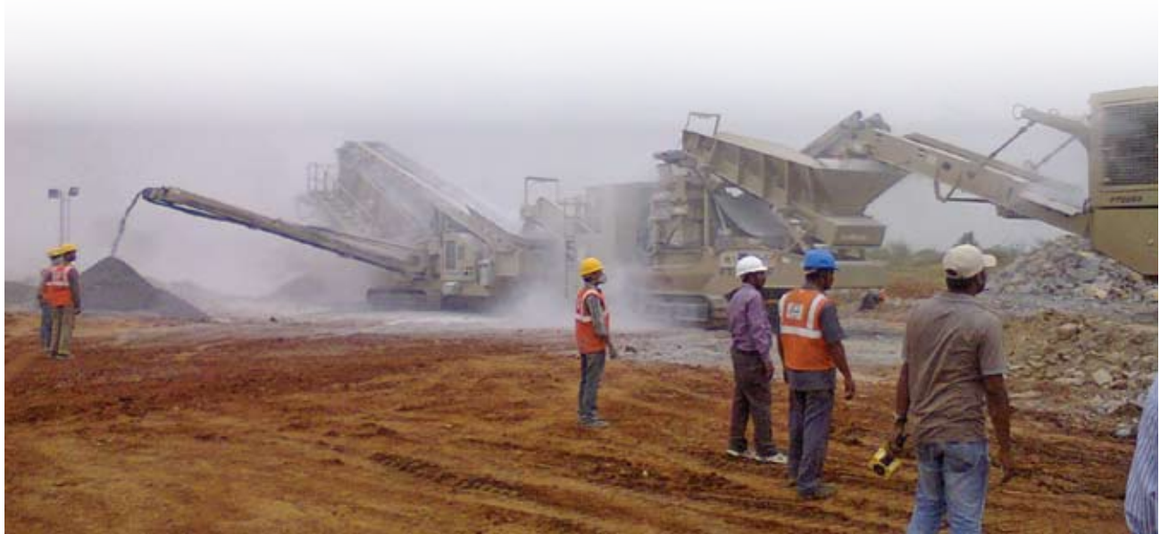
Glimpse of Crushing Plant at Pakur, Jharkhand
